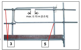
➤ Align the upper railing pipes so that when the rope is swivelled in, it is guided through the aperture.
